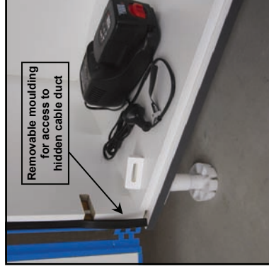
Keep cords tidy in the cable duct
