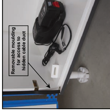
Keep cords tidy in the cable duct
